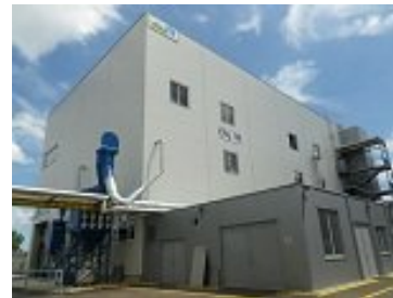
DIC Europe GmbH Vienna Plant
