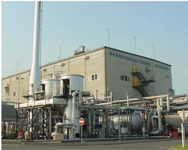
Kashima Plant 1 Ibaraki, Japan
