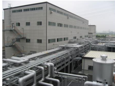
Kashima Plant 3 Ibaraki, Japan
