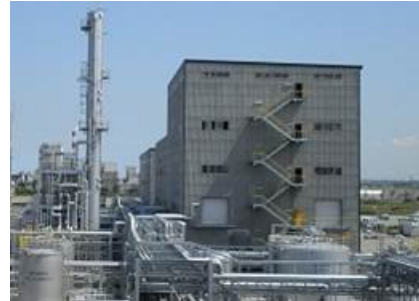
Kashima Plant 4 Ibaraki, Japan
